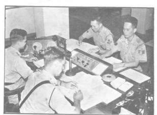
The photographs above show the existing control room and the control table on which the controls for the main, standby and marine G.E.C. sets are located. Additionally, a radio in the form of a telephone set is used.
